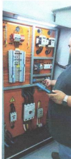
Test e reparos painel geral
